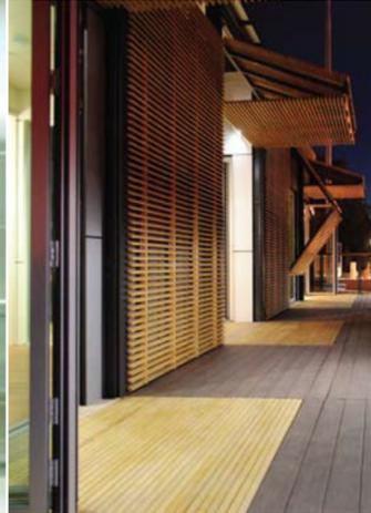
**Figure 197:** RE: FOCUS House. Solar Control Devices, SDE 2010.
