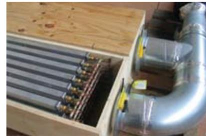
**Figure 211:** Phase Change Material based air tempering system. Detail of the closed ducts system. Napevomo House. SDE
